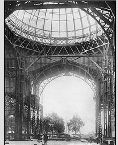
Dome under construction, 1914.
