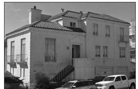
201 Capra Way, still standing as of 2022, and owned and occupied by Ray Martelli.
